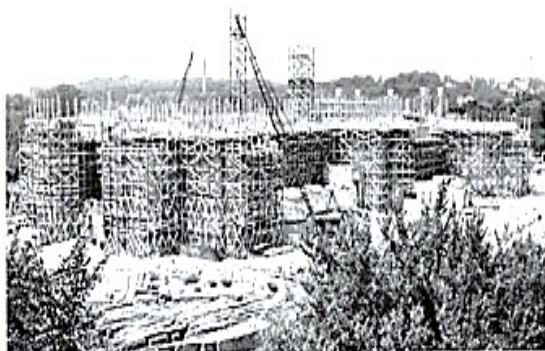
September 23, 1956 — lower part of upper church rises from the scaffolding.
